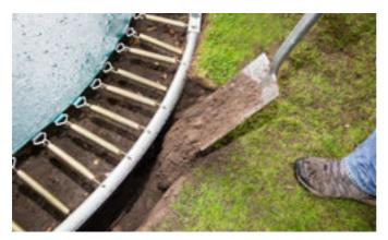
Lift the trampoline into the hole and place on the ledge ensuring the frame is at the correct height. Then back-fill in the gap on the outside of the frame, compact the soil and re-turf.
