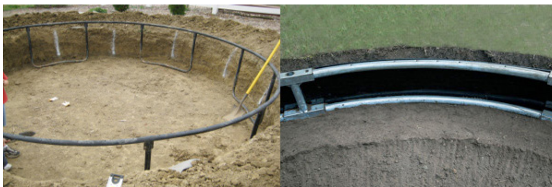
Trampolines sitting in the bottom of the pit can perish quickly (pictured left). Our specifically designed trampolines sit on a ledge with a retaining wall attached to the frame (pictured right).
