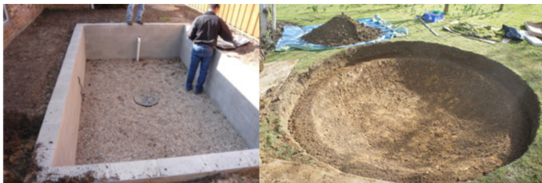
Traditional trampolines are costly to prepare the pit (picture left) compared to the new style in-ground trampolines (picture right).
